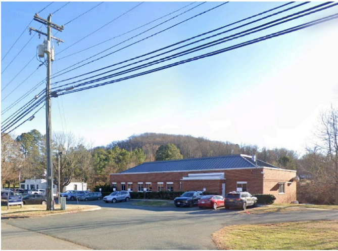
Figure 1: CUAECC building at 2306 Ivy Road – front entrance.
