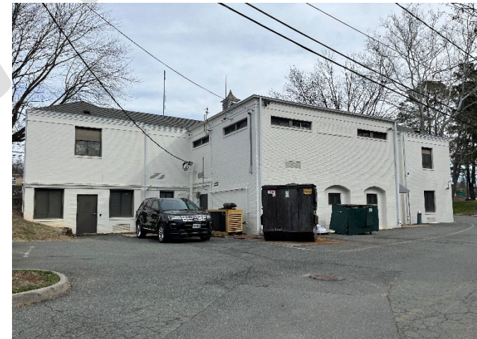
Figure 4: UVA police building at 2304 Ivy Road - back.
