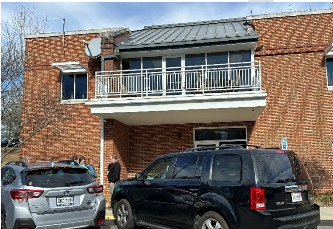
Figure 2: CUAECC building at 2306 Ivy Road - back entrance.
