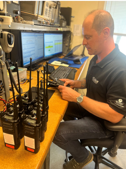
Clear Communications programming radios on the P25 Radio system for 30-day burn in.
